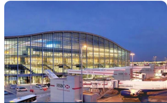
Heathrow Airport, Terminal 5, United Kingdom
