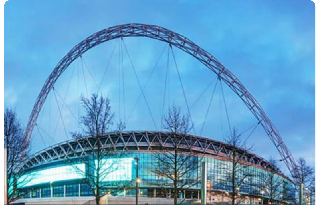
Wembley Stadium, United Kingdom
