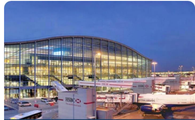
Heathrow Airport, Terminal 5, United Kingdom
