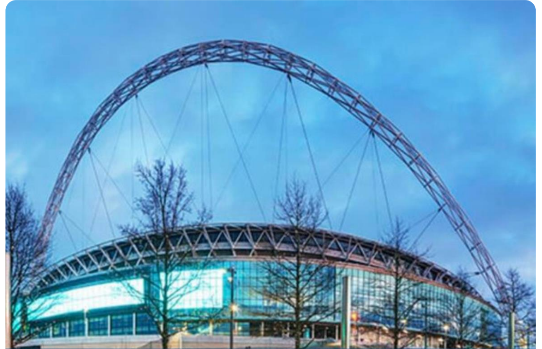
Wembley Stadium, United Kingdom
