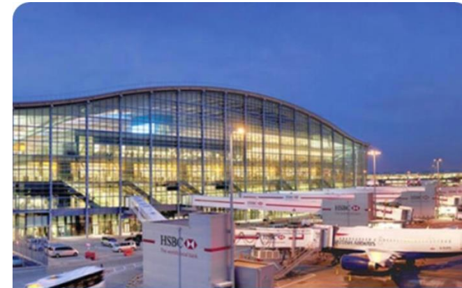
Heathrow Airport, Terminal 5, United Kingdom
