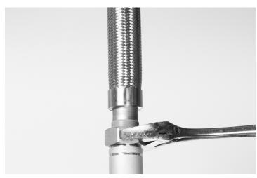
**6.** Bend the flexible hose to achieve the required routing maintaining the minimum bend radius and position the reducer for sprinkler location. When bending the hose allow 65mm of straight hose from the nut, ensure there are no kinks.
