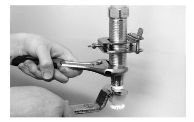
When installing the sprinkler head with a two piece escutcheon, the inner piece should be mounted on the thread of the sprinkler head before attaching to the reducer.
