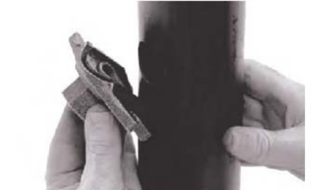
3. Gasket Installation
