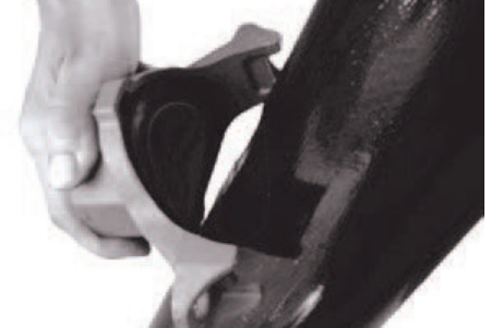
3. Gasket installation
