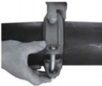
5. Housing Installation
